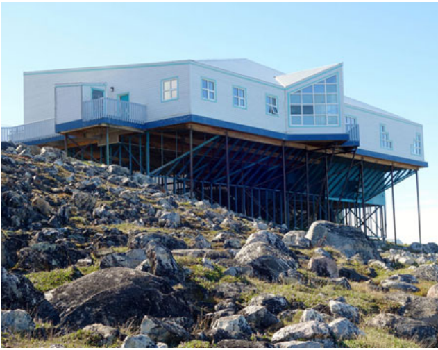
The Pond Inlet Nattinak Visitor Center and Library is built on stilts due to permafrost conditions. (Photo by Jason Little)
